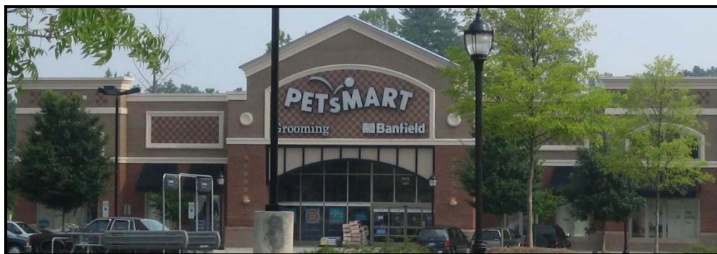
Facade with Recesses & Projections
