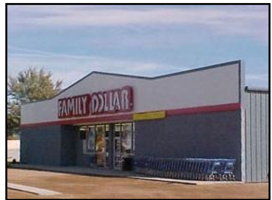
Plain Concrete Block & Metal Façade
