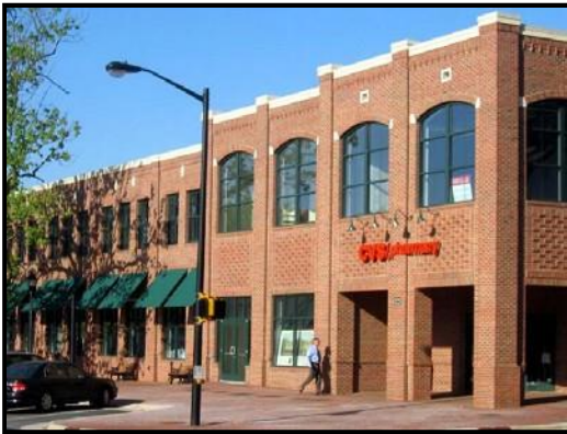
First Floor Windows
