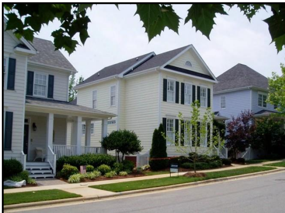
Approximately 12 inch Overhang
