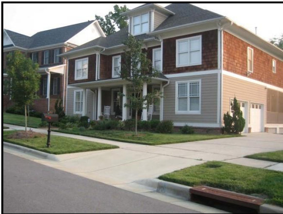
Wood Shingles and Clapboard Siding
